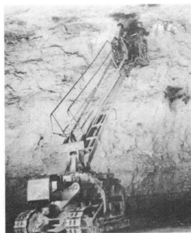
Figure 2. - Traveling crane with self-leveling platform.
