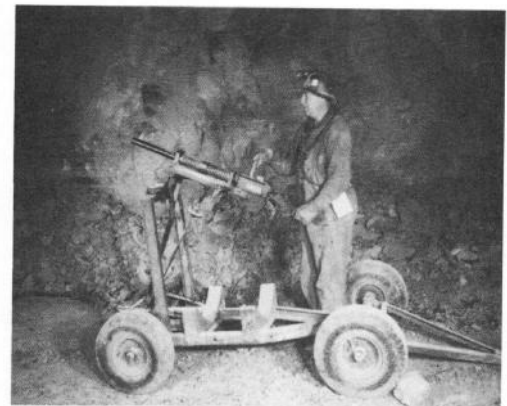
Figure 12. - Industrial gun used for removal of loose rocks on mine walls.
