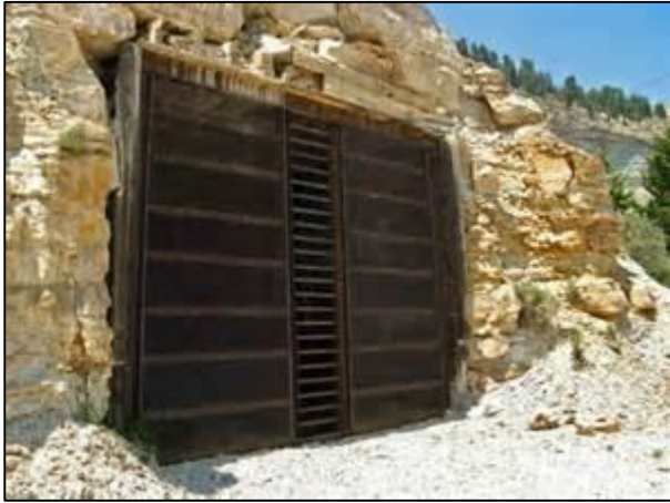
Closed off mine entrance that has a bat gate for bat entry/exit.
