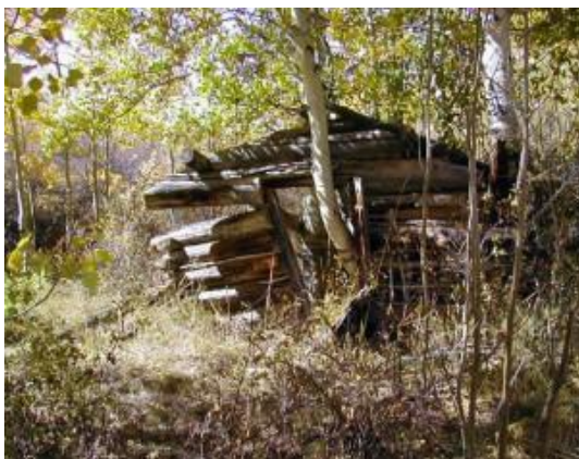
Remains of pump house on top of the mesa
